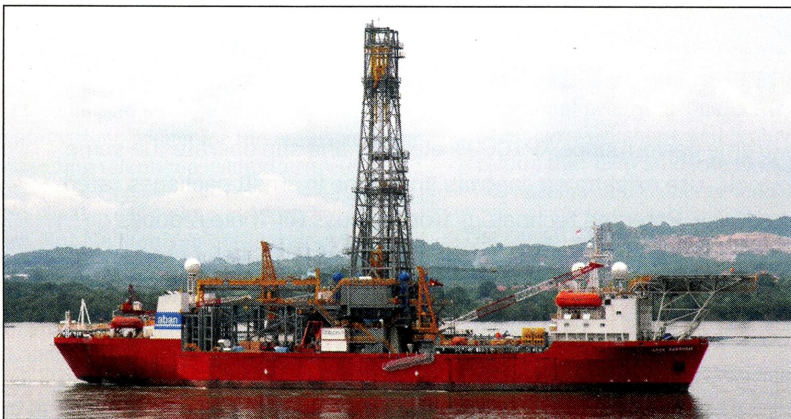
The Aban Abraham underwent major upgrades and has now completed seatrials. It is heading to offshore Africa to drill on the Cape Three Points deepwater block.
